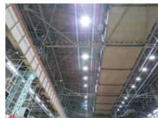
圧造工場に設置したLED照明器具 LED lighting equipment installed in stamping plant
