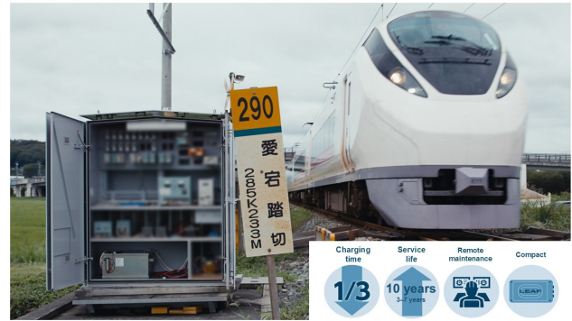
Figure 8 Backup power supply for grade-crossing protection systems (lead-acid battery substitute)
