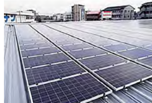
Solar panels are on the roofs of some Kanagawa Nissan dealerships. Power from the panels is supplied to dealerships through the PPS system.
