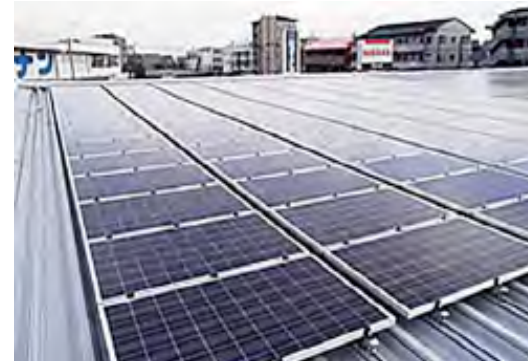
Solar panels on the roofs of some Kanagawa Nissan dealerships. Power from the panels is supplied to dealerships through the Nissan PPS system.
