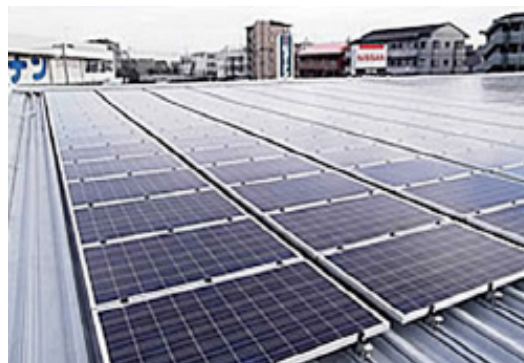
Solar panels are on the roofs of some Kanagawa Nissan dealerships. Power from the panels is supplied to dealerships through the PPS system.
