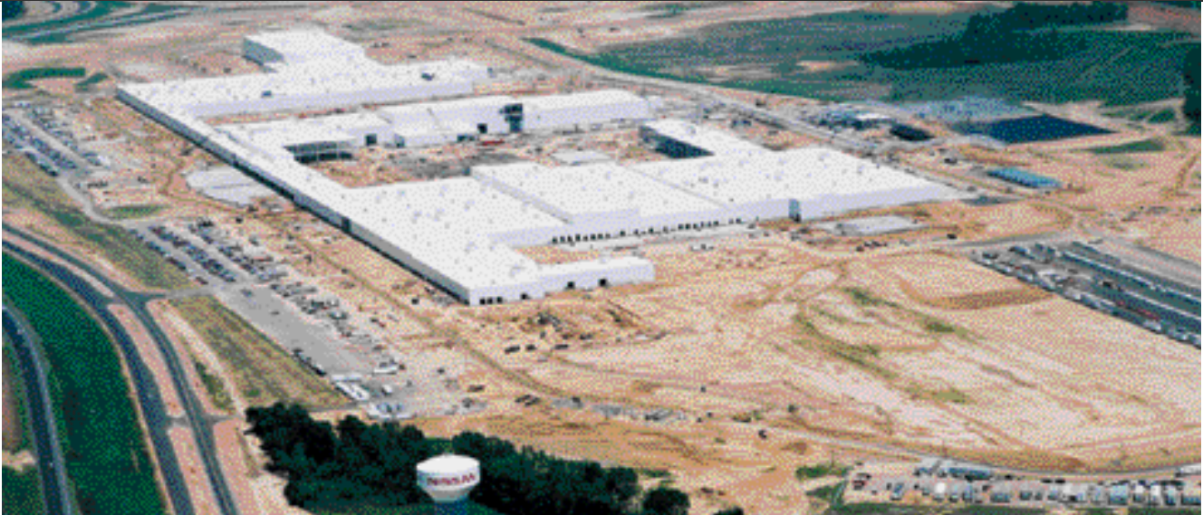
Construction at Nissan's new Canton, Mississippi plant; production is scheduled to begin in 2003
