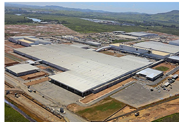
The new Resende Plant, to be surrounded by a "Green Belt" that helps absorb CO 2 and reduces noise levels.
