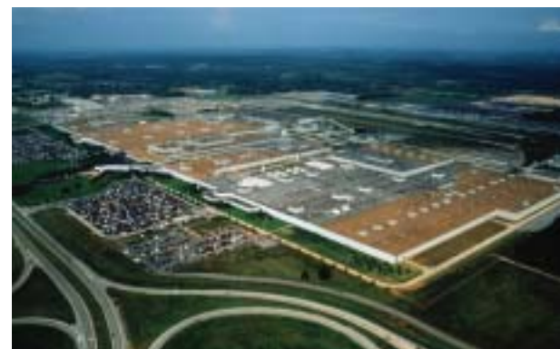
Nissan's Smyrna plant, Tennessee
