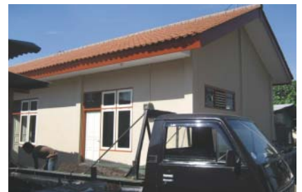
Nissan aided in the reconstruction of this elementary school in Indonesia
