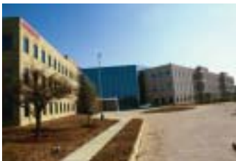
New NMAC Customer Service Center, Texas
